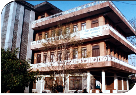
First Administrative Office
